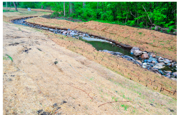
Figure 4. Area with live stakes along County Farm Drain, Spring 2012. Photo by Dan Bruell, used with permission.
